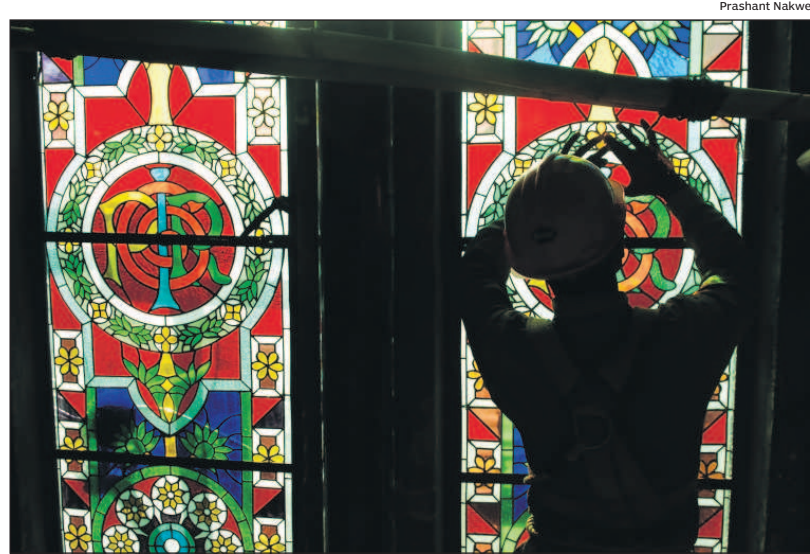
WORLD-CLASS VISION: A worker renovates the CST dome
